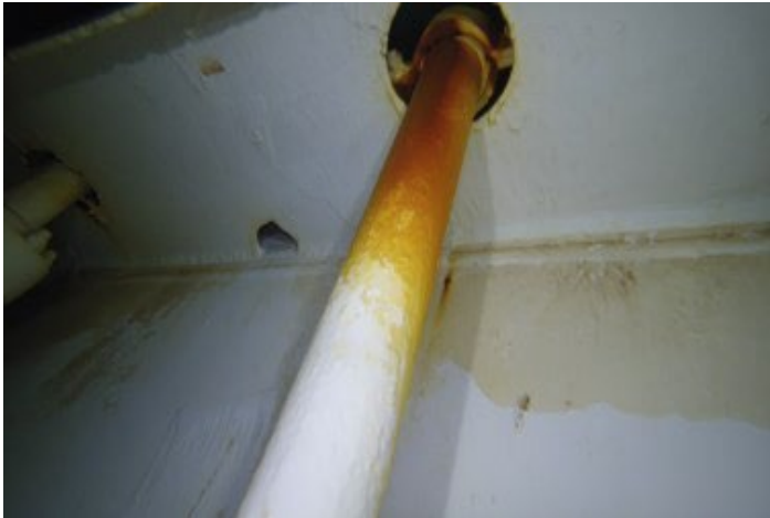
Sounding Tube Coating Failures
