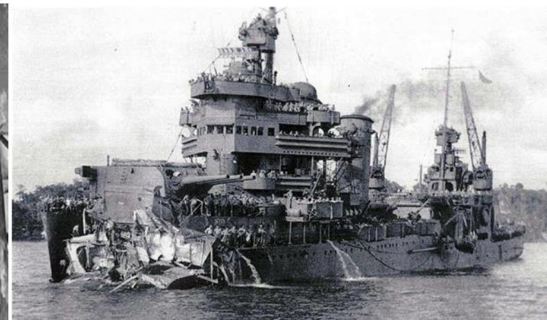
The USS New Orleans (CA-32) after a torpedo blew off her bow on 30 Nov 42. The torpedo detonated the forward magazines and destroyed 150 feet of hull. A further 50-yard length of the ship's bow and forecastle tore away from the ship as she struggled to stay afloat.
