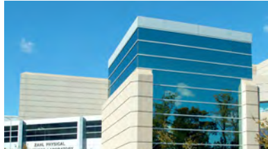
Open areas for researchers and access to existing facilities
