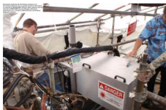
VLS Tube Repair NAVSEA PH Shipyard
