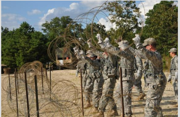
Install Wire Obstacle
