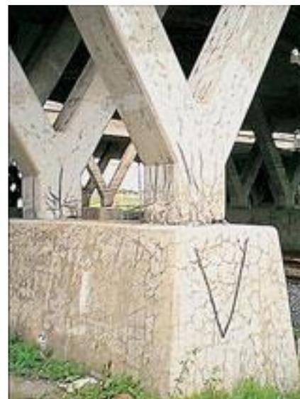
Alkali-Silica Reaction in Concrete
