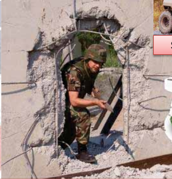
High explosive ammunition creating an opening in a double reinforced concrete wall through which infantry can pass.
